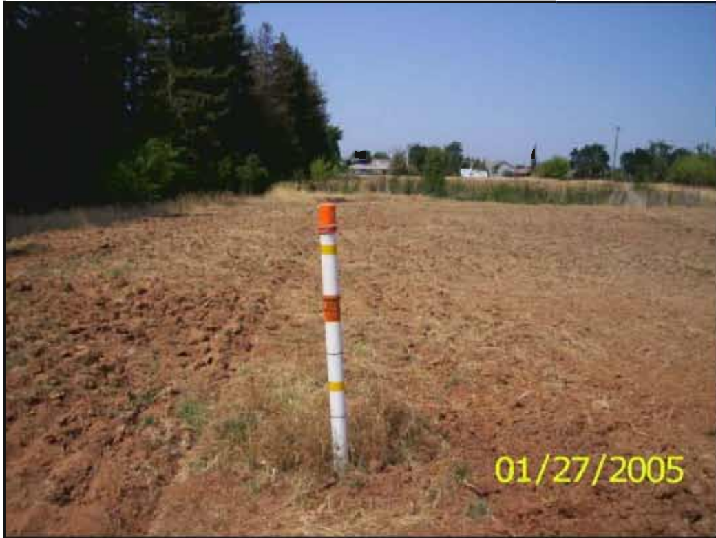
Photograph 1: Example of Electrolysis Test Station.
