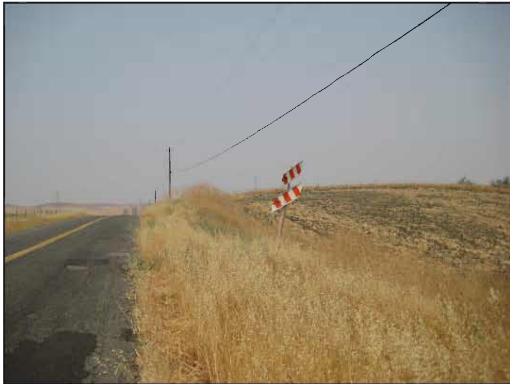
Photograph 2: Example of Pipeline Marker.
